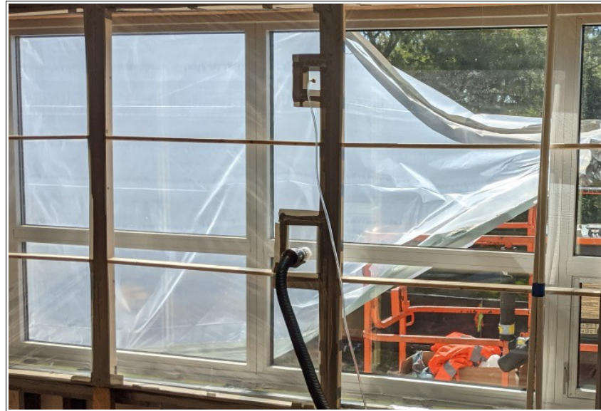
Fig. 01: Tare Sheet Removal – Framed Window Opening
